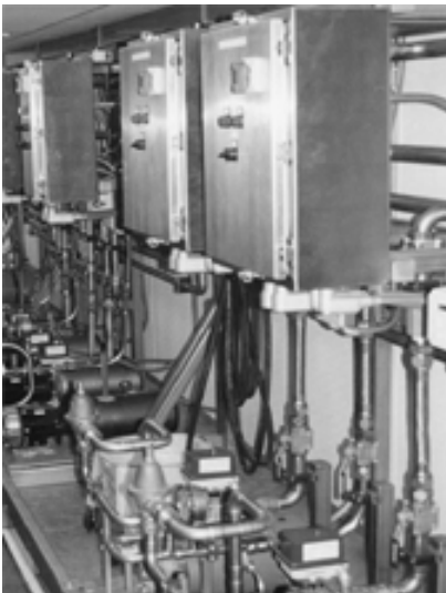
The NOxOUT ULTRA SCR system
