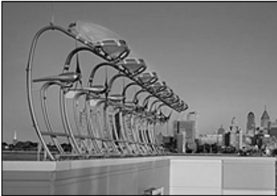
Modular wind turbine system installed on a parapet
