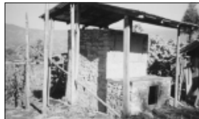
Figure 5: Improved cardamom dryer Model-2
