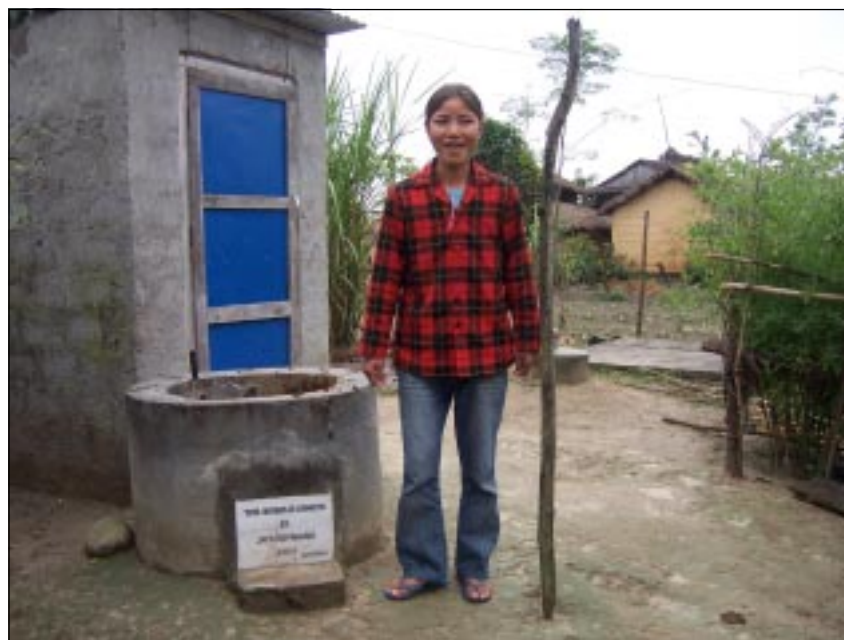
Figure 4: A toilet connected to a mini biogas plant
